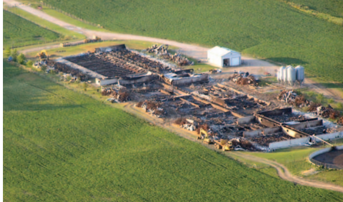
Figure 1.0. This large swine barn was completely destroyed by fire. (Photo credit: P. Stolk, Farm Mutual Reinsurance Plan)
